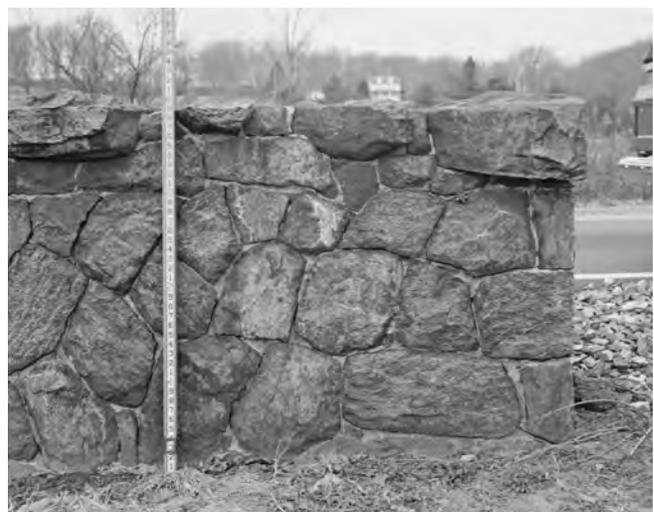
*Example: A wall with mortar added for stability showing preferred deep raking of the mortar in the joints.*
